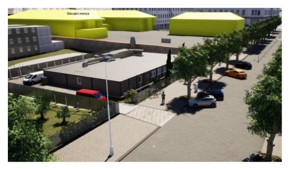
The temporary canteen will take a form of a single-storey building consisting of several interconnected cells. This solution is both very economical and flexible to adjustments. Moreover, the actual construction is simple and fast without major demands for the site preparation.
